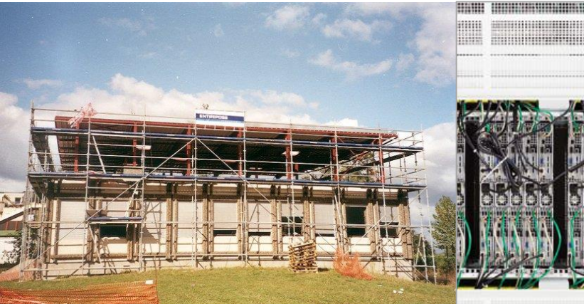
The new Data Center
